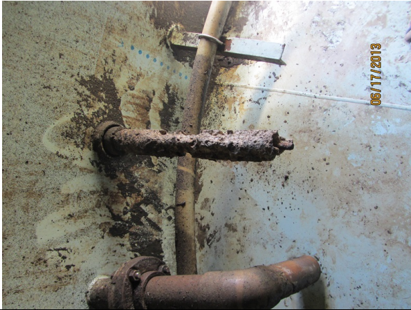
Water Tank -- Tank Anode
