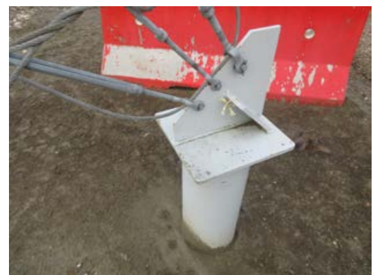
Guy Wire turnbuckles and support
