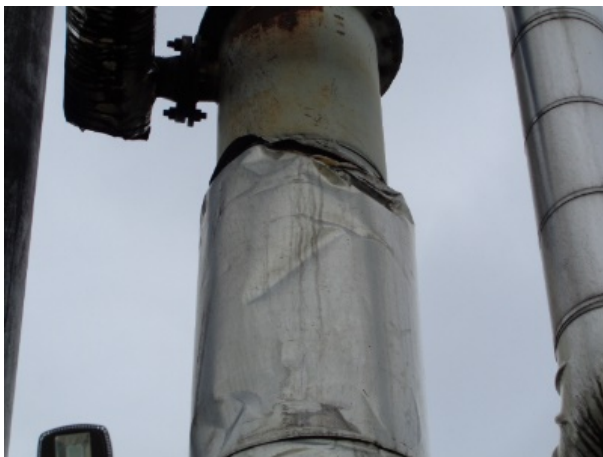
DISTILL COLUMN CLADDING DAMAGE
