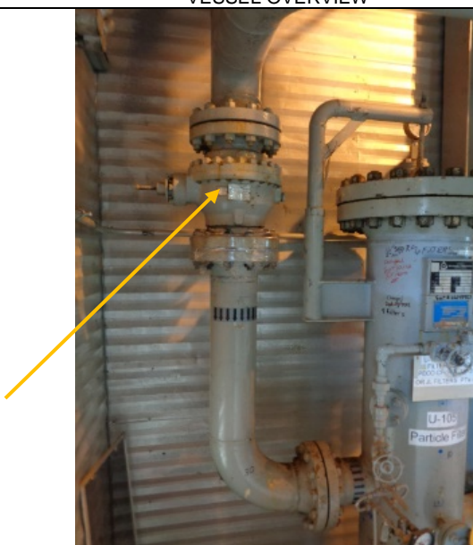
UNLOCKED OPEN VALVE BETWEEN FILTER AND UPSTREAM PSV OFF OF INLET SEP.
