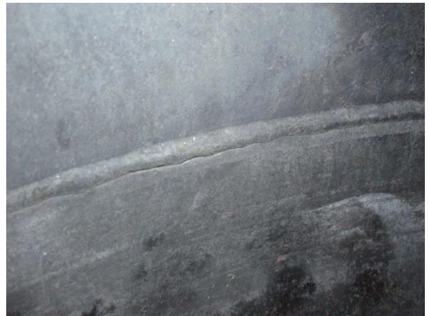
Bottom head to shell circ weld
