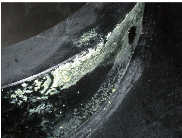
Some waxy deposits remaining on manway nozzle
