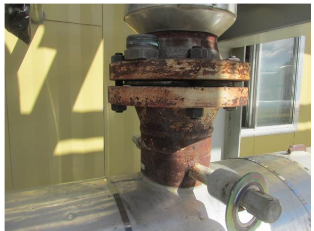
Nozzle paint deterioration due to heat, no significant corrosion
