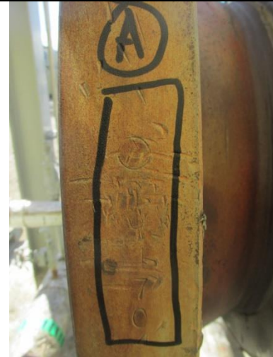
A# stamped in shell flange
