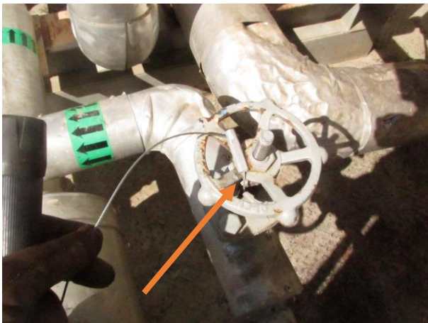
Tube side PSV outlet isolation valve carsealed open
