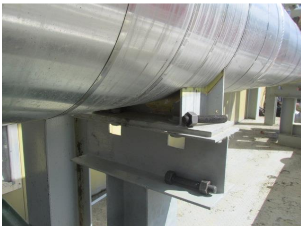
Saddle supports bolted to beams
