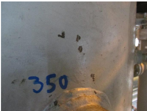
Minor paint damage to shell
