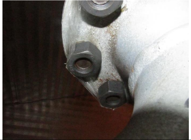
PSV inlet flange shortbolting bottom of studs
