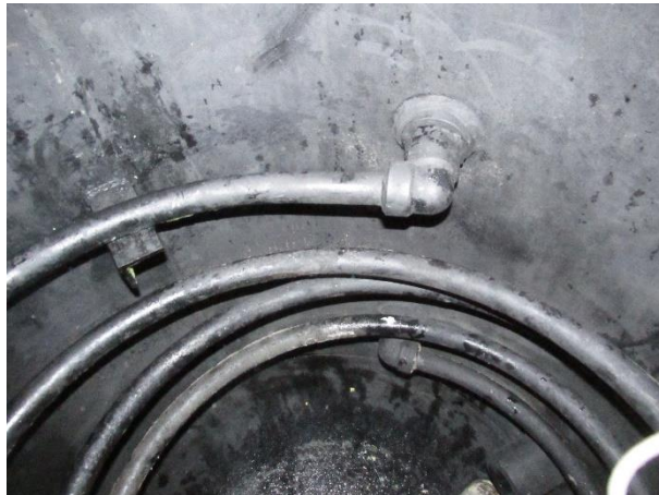
Internal coil attachment and supports
