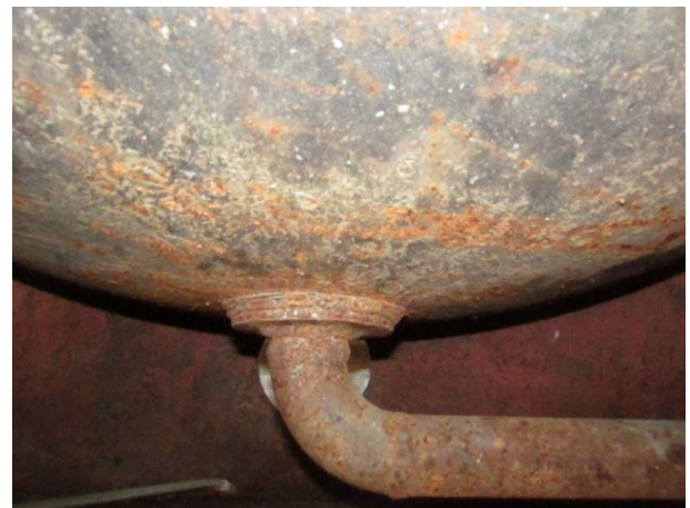
Bottom head general corrosion
