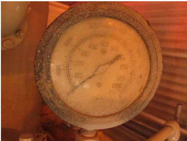
Paint overspray on bridge PSI gauge glass
