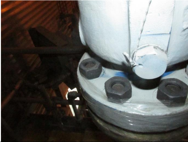
PSV inlet flange shortbolting top of studs
