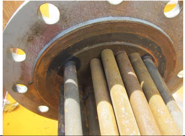
Tube to tubesheet
