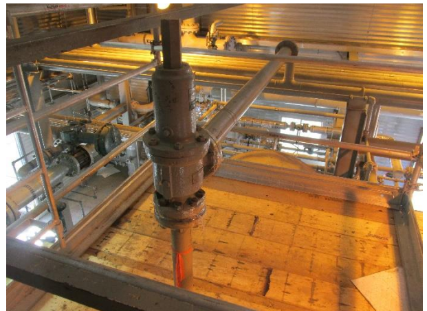
Shell side PSV off stabilizer feed drum
