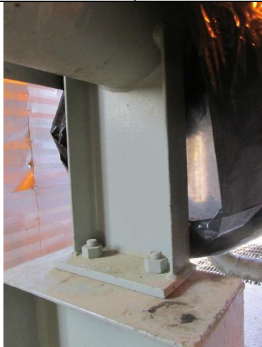
Saddle supports, seal welded, bolted to Beam
