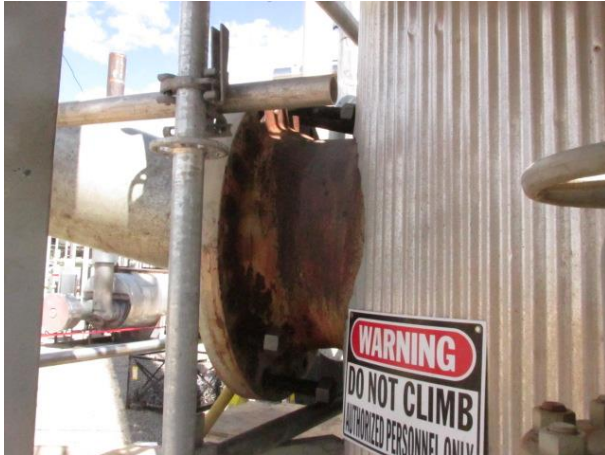
Paint deterioration on bottom manway
