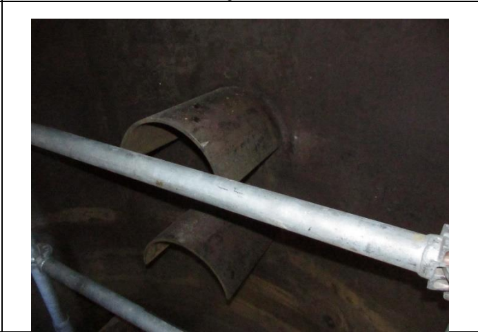
Nozzle cover attachments
