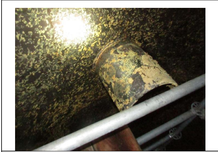
Top shell nozzle cover attachment
