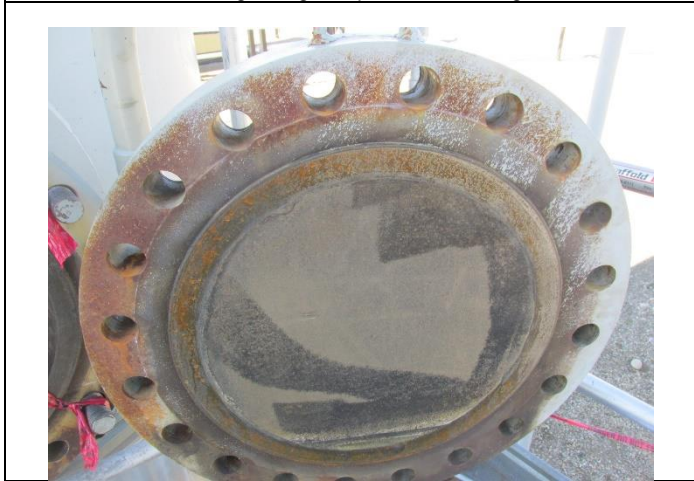
Manway internal surface
