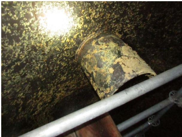
Top shell nozzle cover attachment
