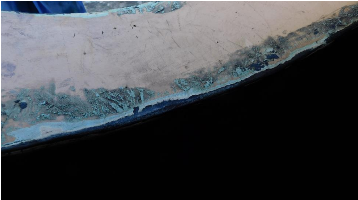
Photograph 21: Coating Failures on Entrance Manway
