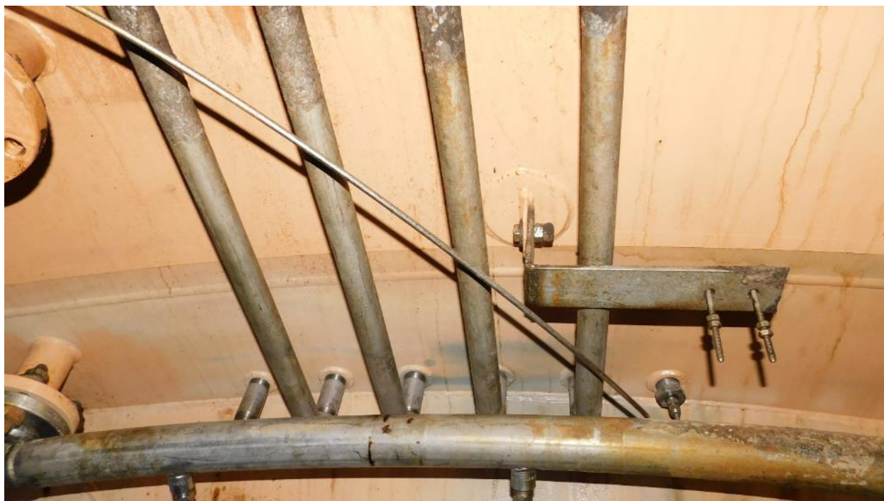
Photograph 31: Internal Nozzles
