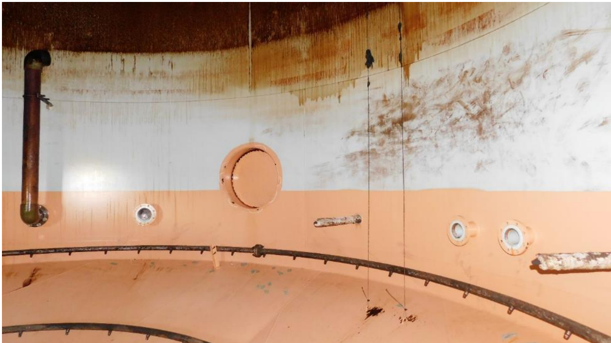
Photograph 19: Internal Nozzles
