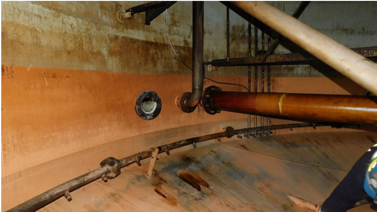
Photograph 20: Internal Nozzles
