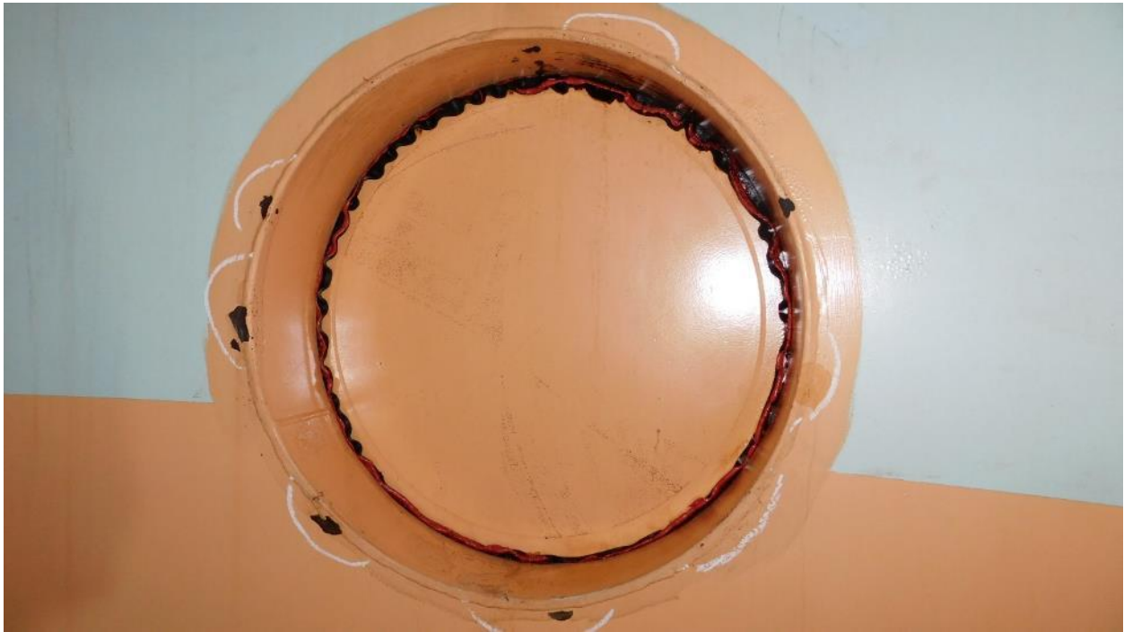
Photograph 28: Coating Failures Around Internal Manway
