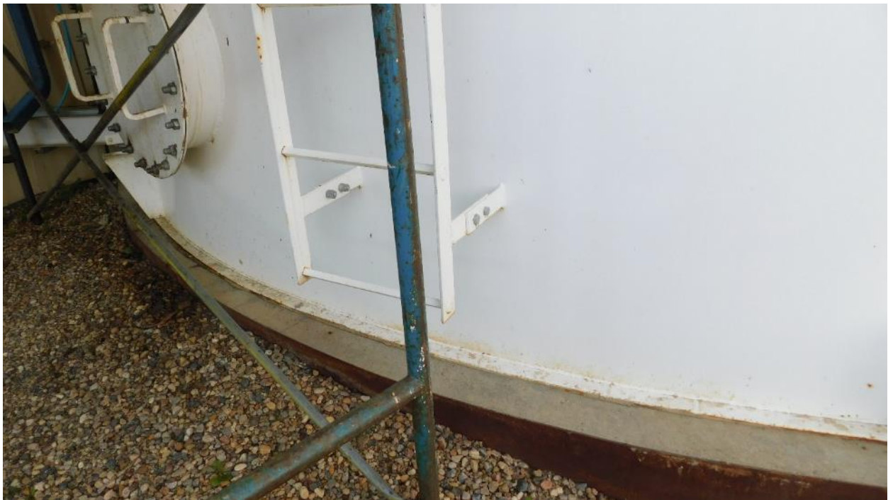
Photograph 7: Foundation Concrete Ring Wall
