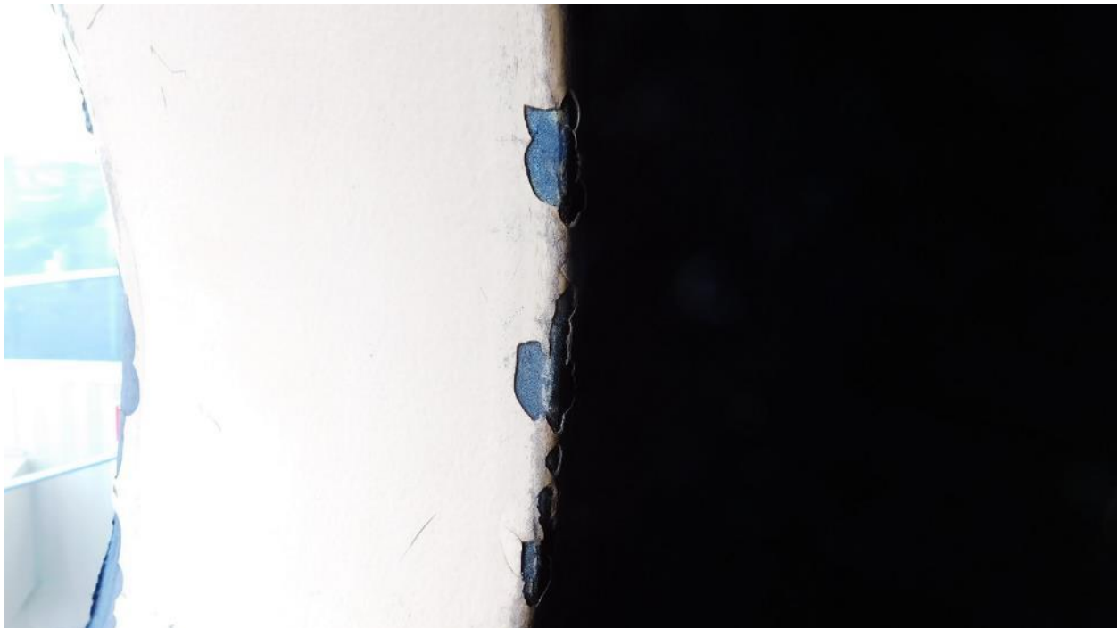
Photograph 27: Coating Failure on Manway
