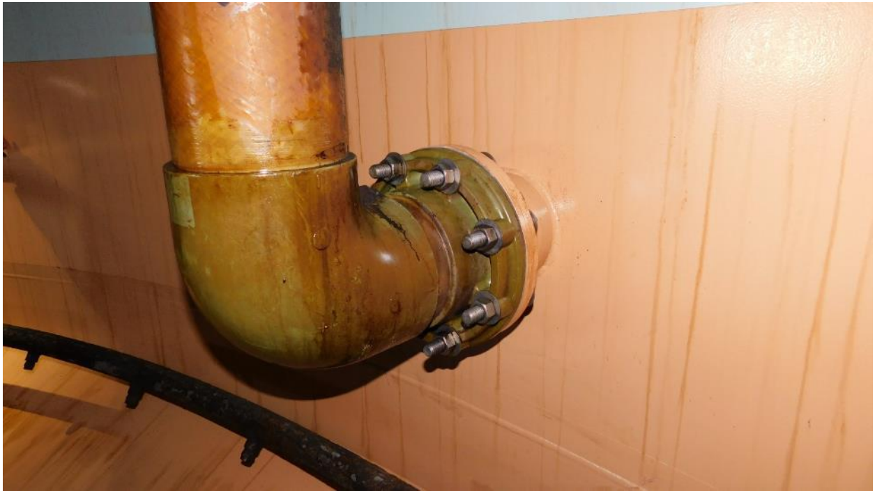
Photograph 32: Internal Nozzle
