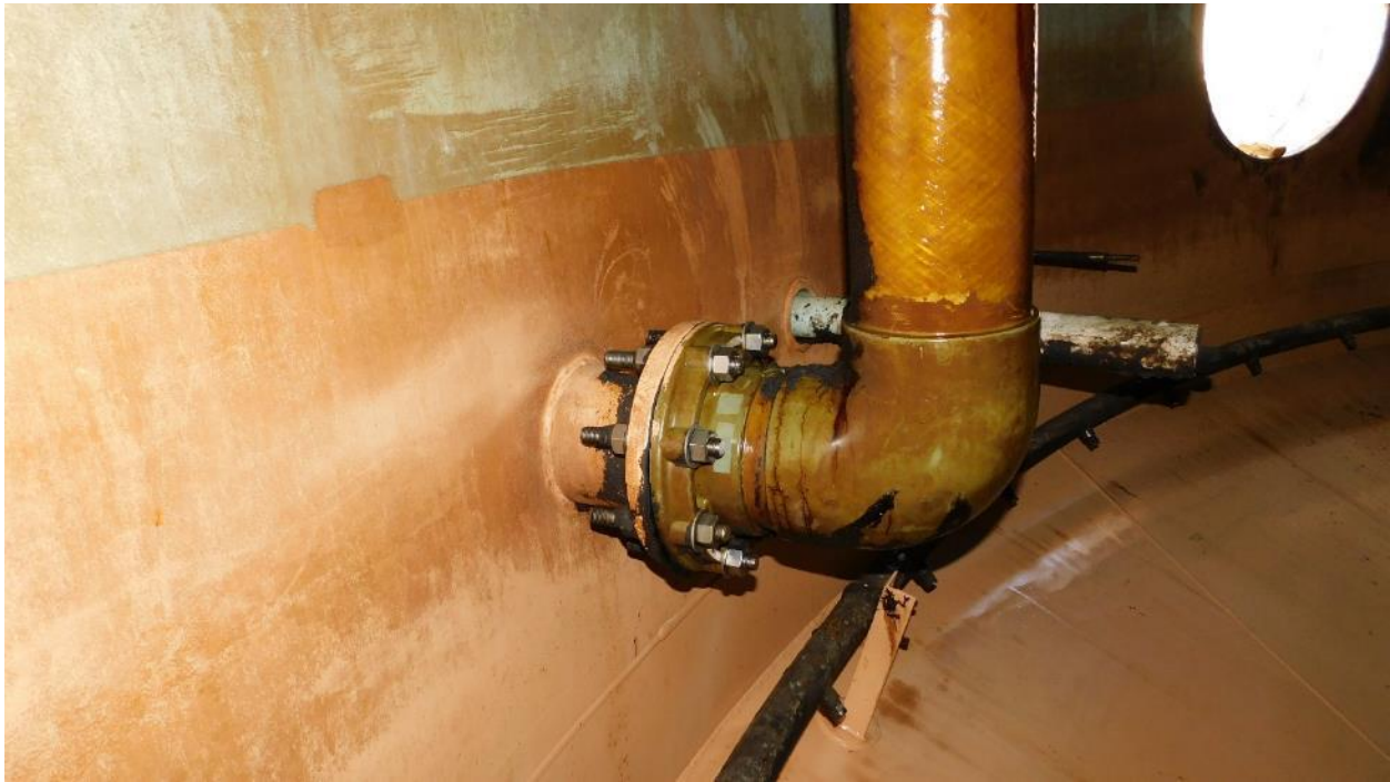
Photograph 24: Internal Nozzle
