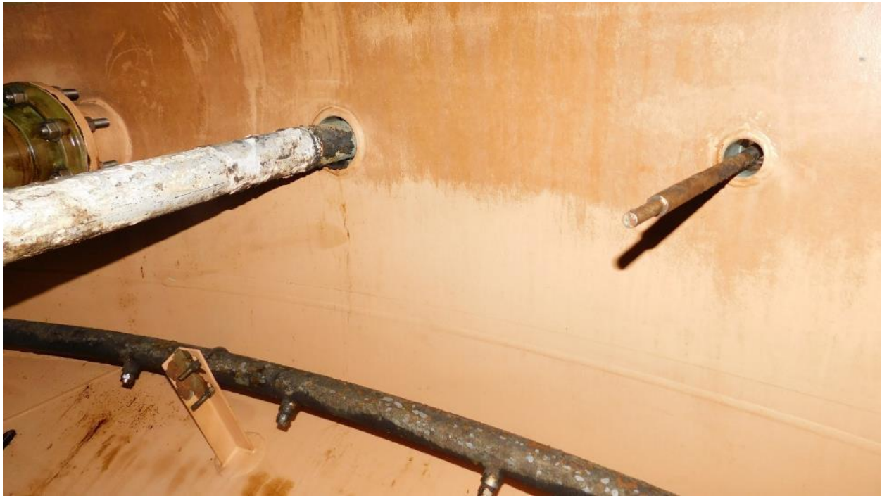
Photograph 26: Anode and Temperature Probe
