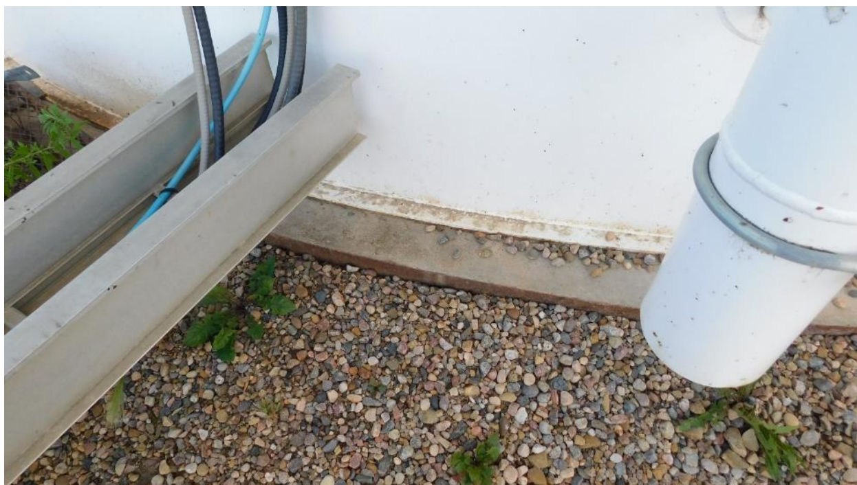
Photograph 8: Foundation Concrete Ring Wall
