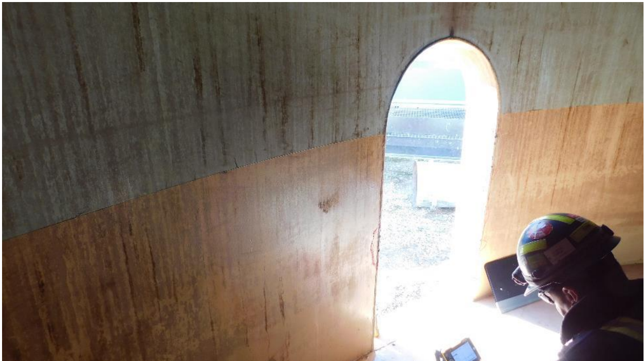
Photograph 28: Internal View of Entrance Manway
