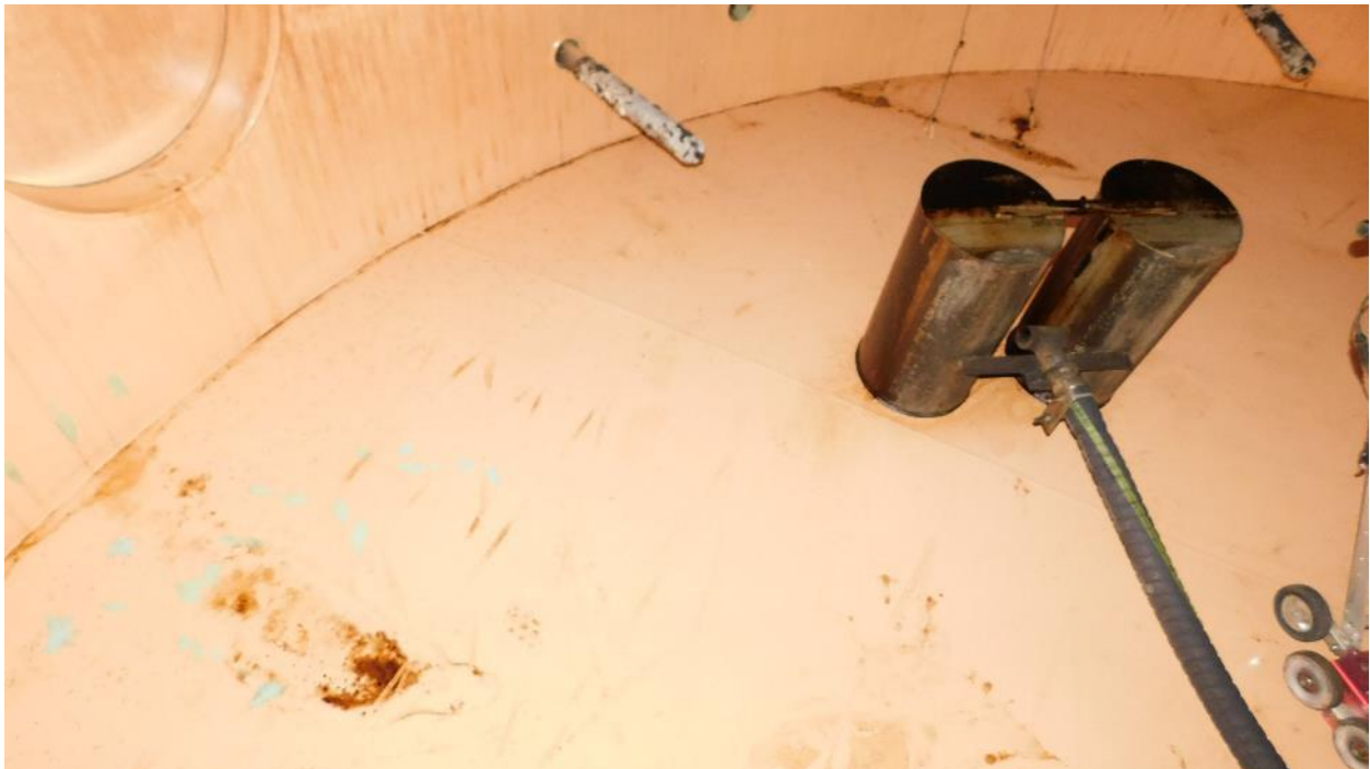
Photograph 14: Bottom Plate Overview
