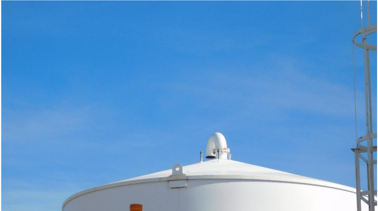
Photograph 34: External Fixed Roof
