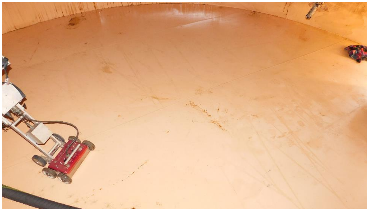
Photograph 10: Bottom Plate Overview
