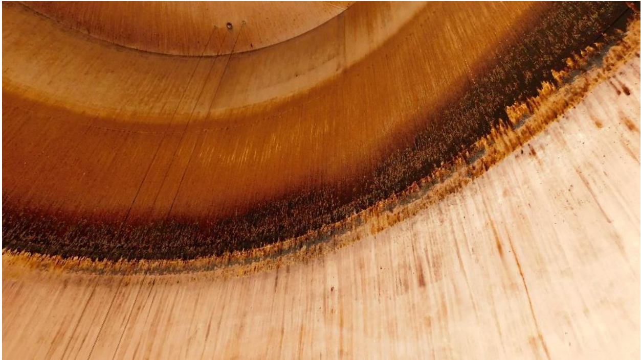
Photograph 15: Internal Shell Plate Overview
