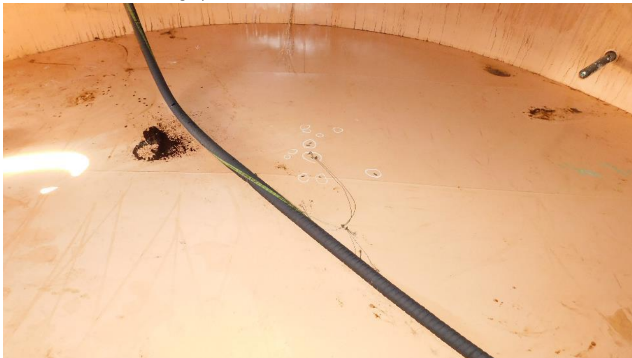
Photograph 9: Bottom Plate Overview
