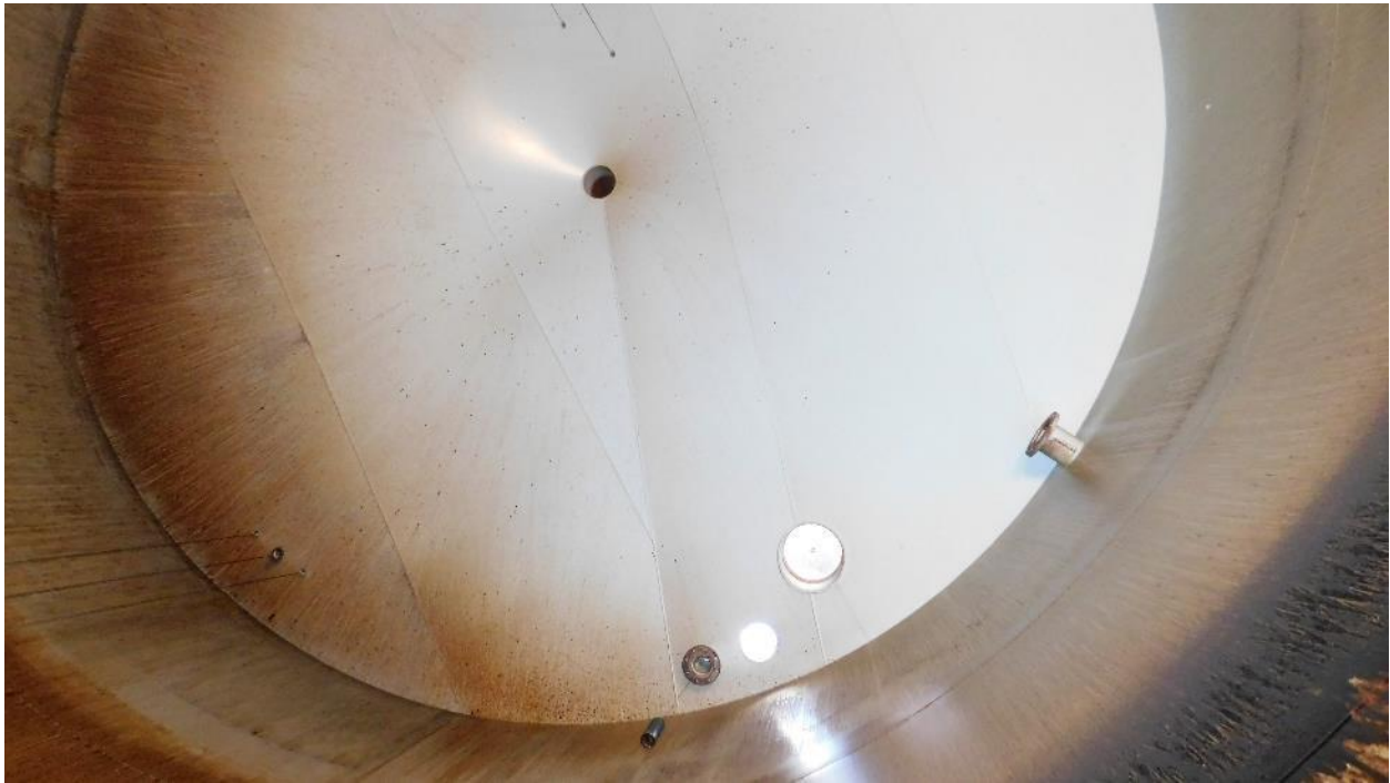
Photograph 33: Fixed Roof Internal Surface
