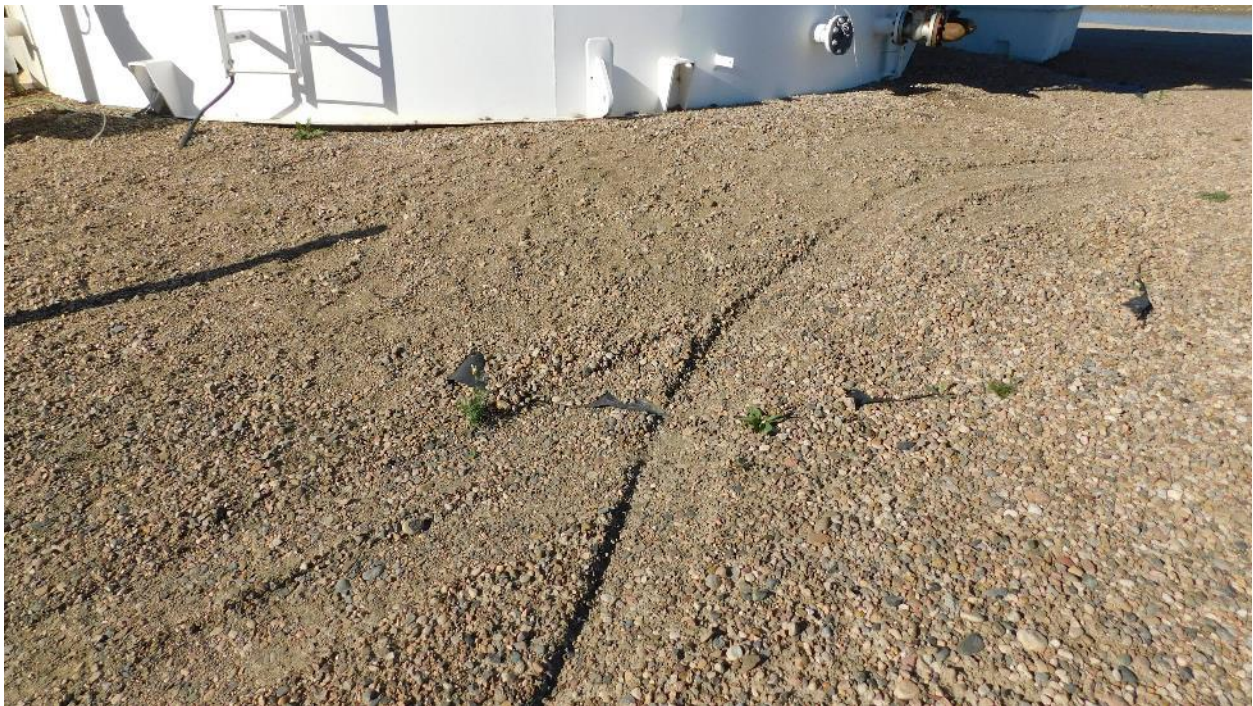
Photograph 8: Foundation Material (Gravel)
