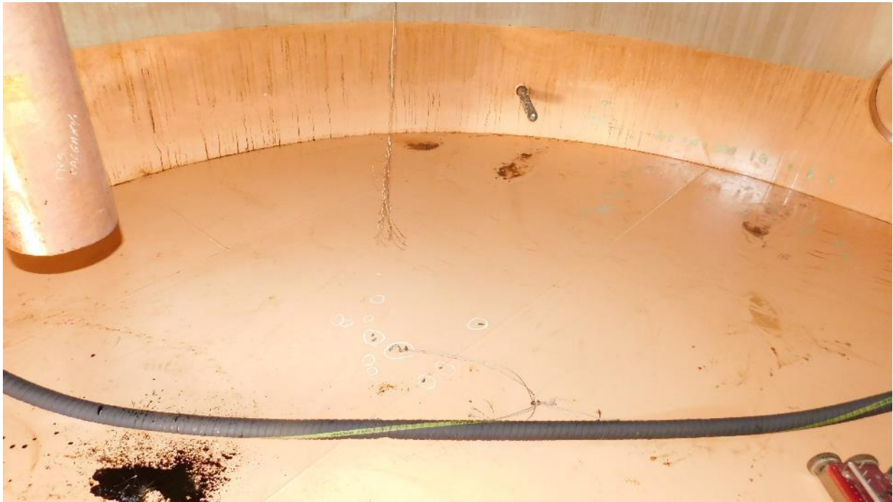
Photograph 11: Bottom Plate Overview
