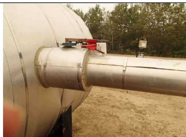
The valve on the outlet of the vessel going to the flare which is car-sealed open in normal operation.
