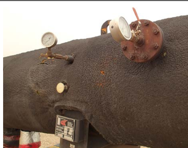
The two pressure gauges and one temperature gauge that need replaced.
