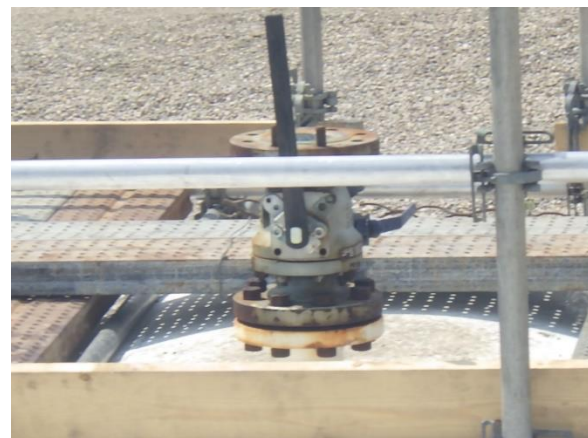
WEST PSV ISOLATION VALVE (PSV OUT FOR SERVICING)
