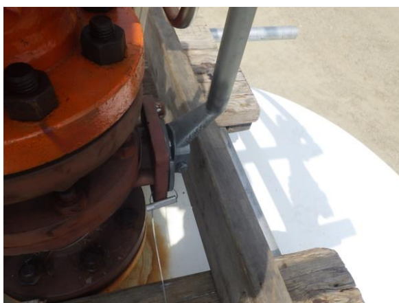
EAST PSV ISOLATION VALVE (CARSEALED OPEN)
