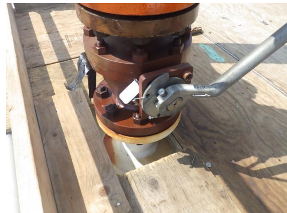
MIDDLE PSV ISOLATION VALVE (CARSEALED OPEN)
