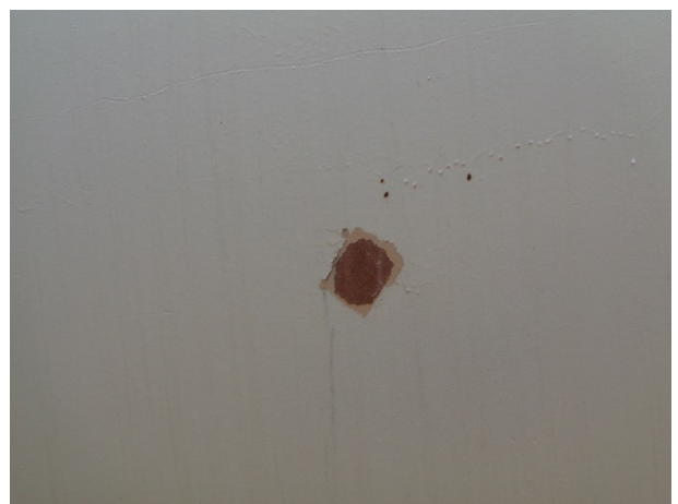
Shell paint deterioration to bare steel
