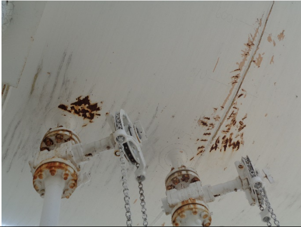
BOTTOM SHELL COATING DAMAGE, MINOR RUSTING
