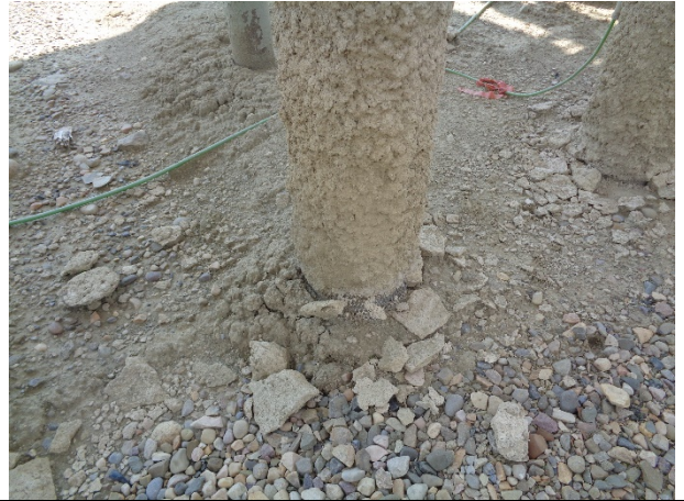
MINOR FIREPROOFING DAMAGE AT BASE OF SUPPORTS
