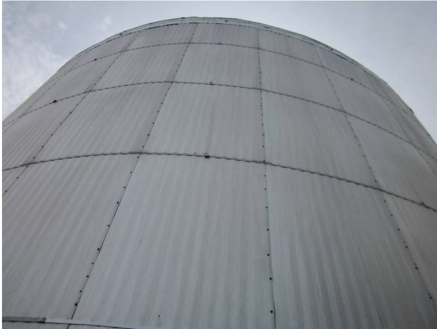
Photograph #27: Insulated Shell Plate
