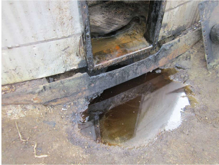
Photograph #26: Void Beneath Manway from Cleaning
