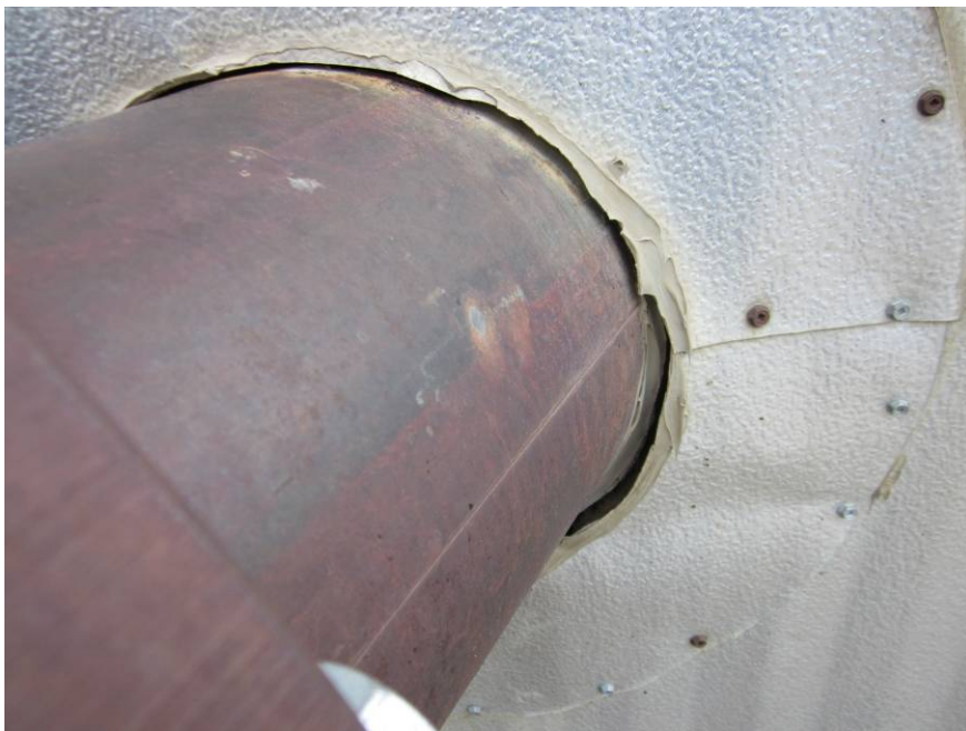
Photograph #28: Sealant Failures
