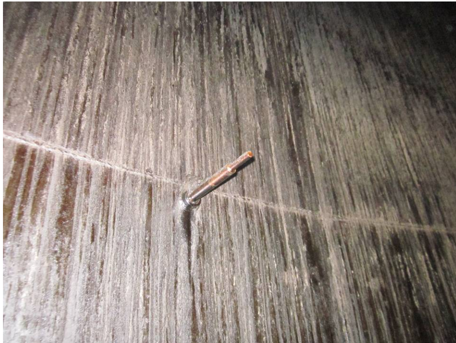
Photograph #44: Temperature Probe
