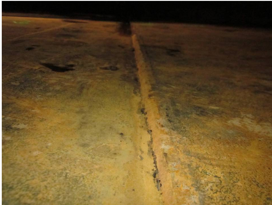
Photograph #10: Lap Welded Bottom Plate
