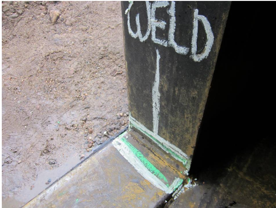
Photograph #48: Manway Weld Repair
