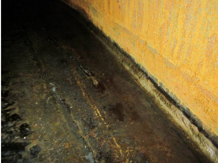
Photograph #6: Internal Shell-to-Bottom Weld
