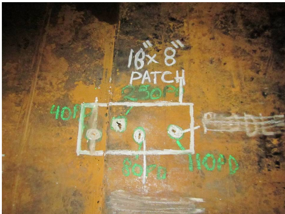
Photograph #17:18 * 8 inch Recommended Patch
