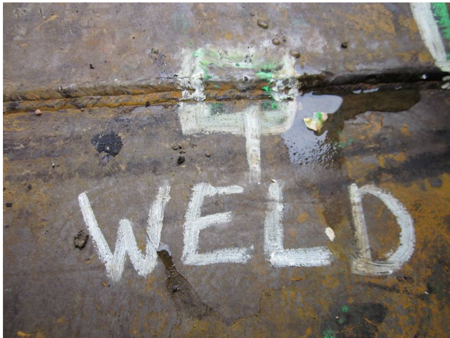
Photograph #47: Manway Weld Repair
