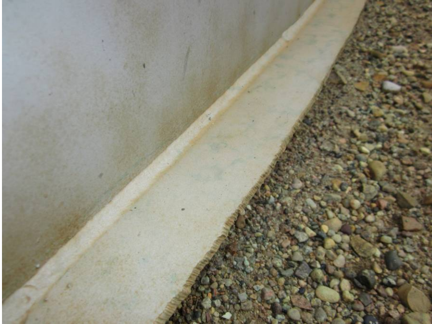
Photograph #6: External Shell-to-Bottom Weld
