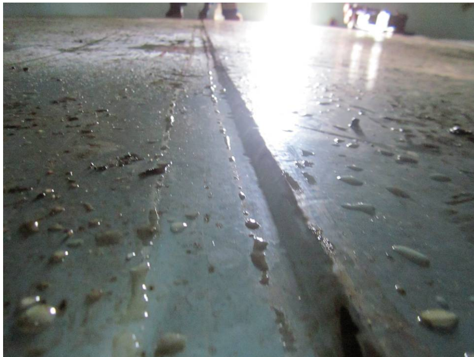
Photograph #11:Lap Welded Bottom Plate
