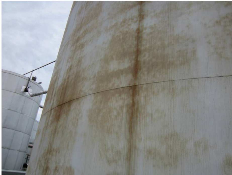
Photograph #19:Oxidation on Shell Plate
