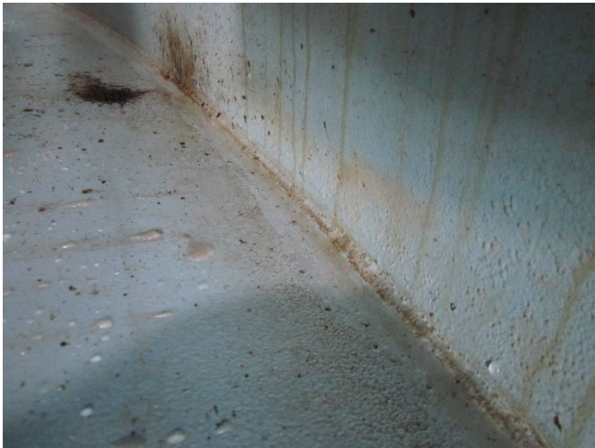
Photograph #7: Internal Shell-to-Bottom Weld
