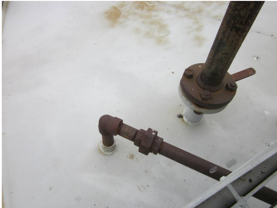
Photograph #42:Roof Nozzles
