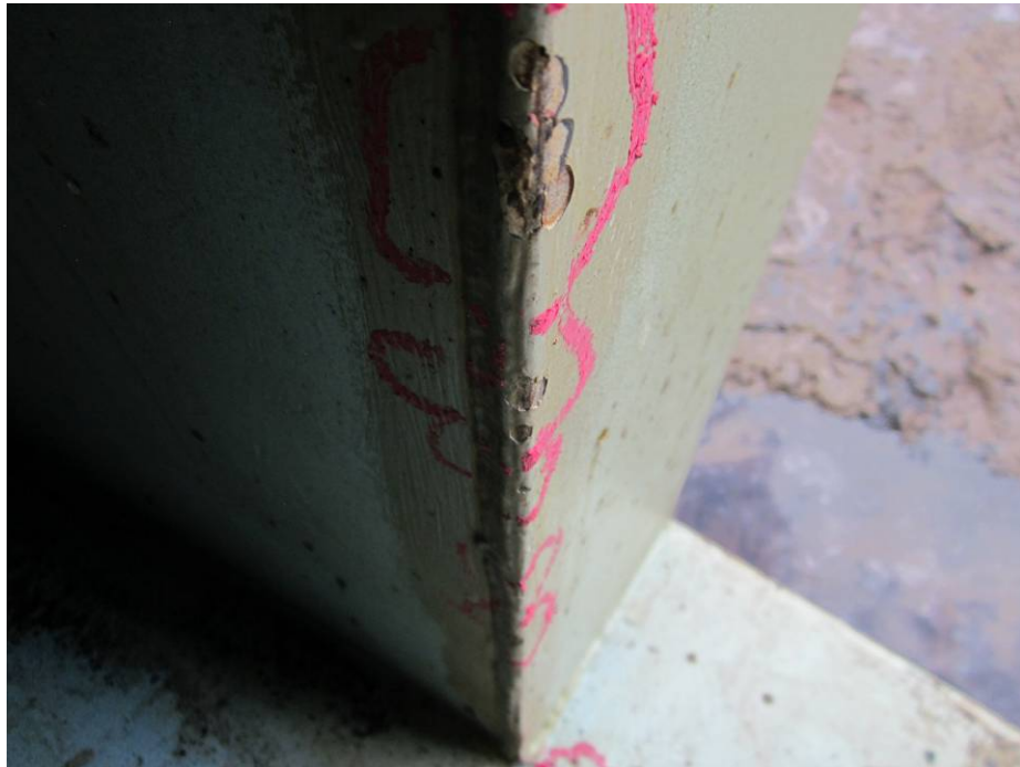
Photograph #31: Coating Failures on Manway
