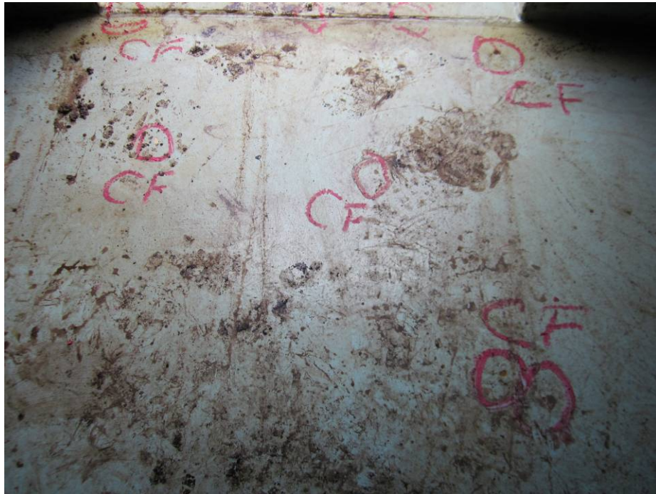
Photograph #12: Coating Failures
