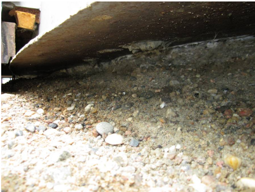
Photograph #16:Void Beneath Tank
