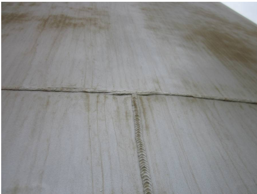
Photograph #18: Butt Welded Shell Plate
