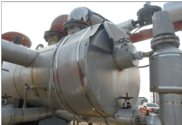
DAMAGED INSULATION
