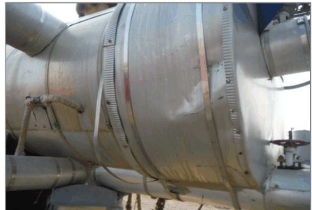
DAMAGED INSULATION
