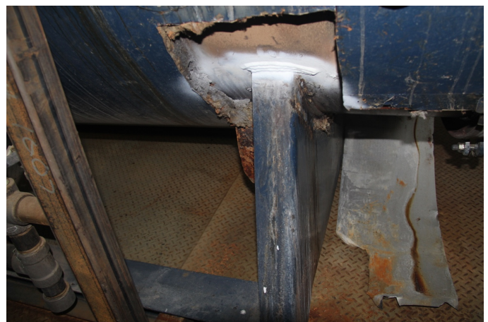
Missing Insulation and loose cladding
