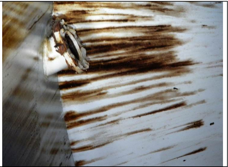
COATING PEELING ON UPPER SHELL NOZZLE
