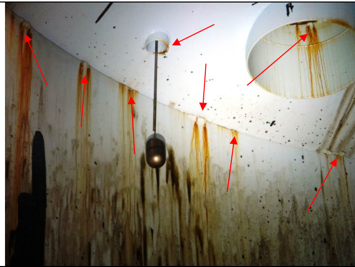
COATING PEELING AT THE ROOF TO SHELL INTERFACE
