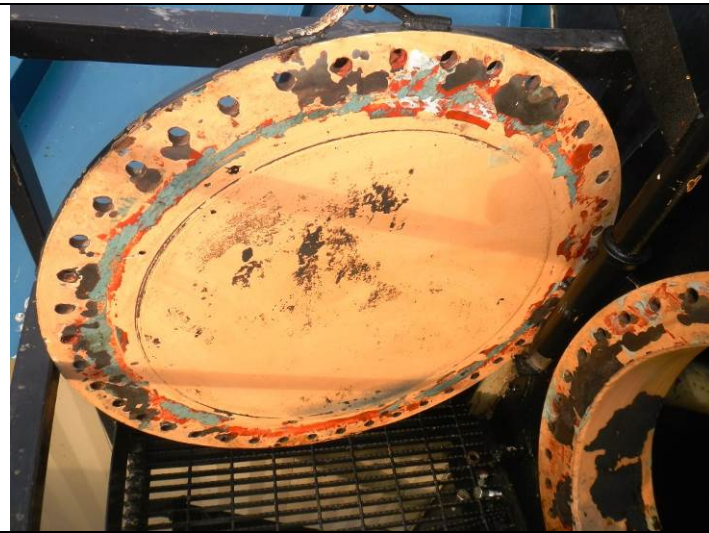
COATING IN POOR CONDITION ON MANWAY COVER
