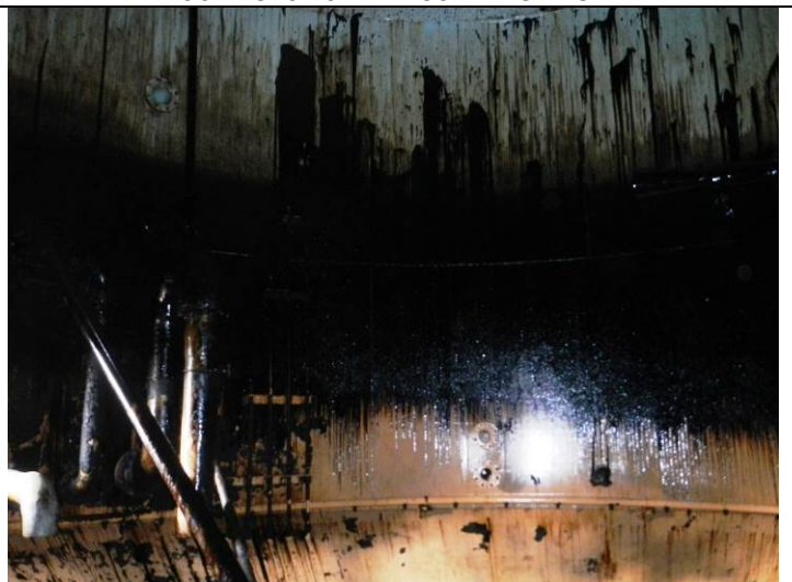
OILY RESIDUES AND SCALE BUILT UP ON SHELL
