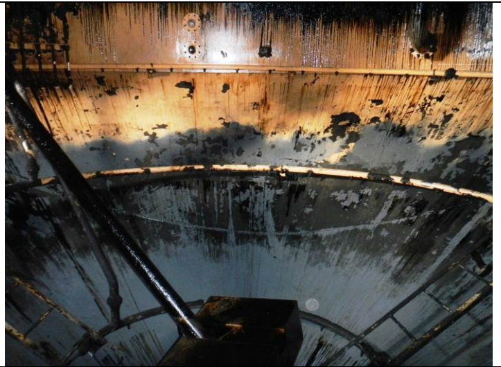
CONE SECTION AND SCALE BUILT UP
