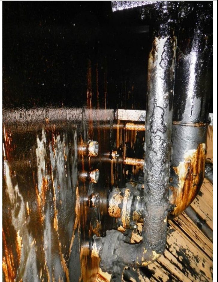
SCALE BUILT UP ON RISERS
