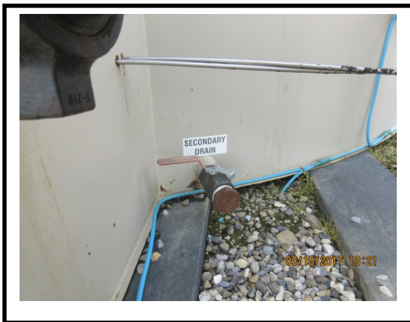
External shell supported on planking & grounding in place.
