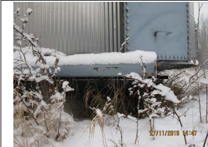
TANK SKID SET ON PILES ABOVE GROUND
