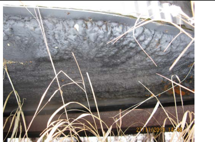
UNDERSIDE OF TANK WITH SPRAY FOAM INSULATION LIQUID.
