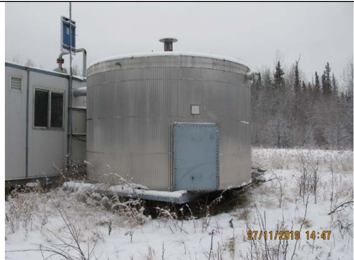
OVERALL VIEW OF TANK SET ON PILES
