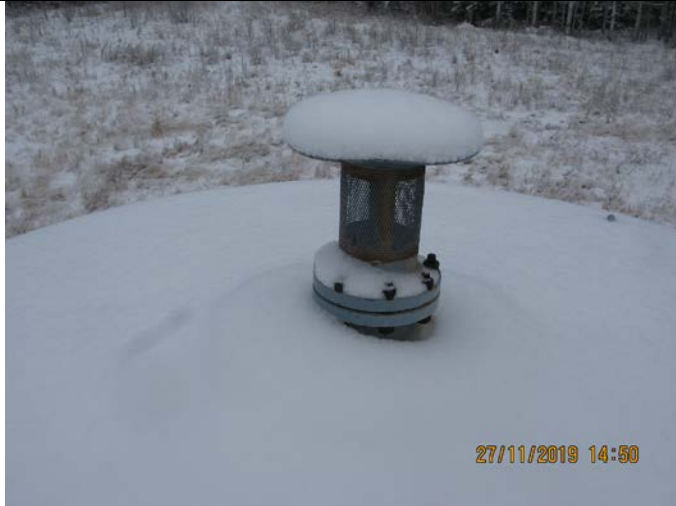
TANK VENT ON TOP OF TANK WITH BIRD CAGE
