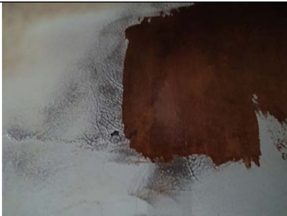
The patch that was applied to the north side of the vessel, cracking to the coating can be seen beside the patch.
