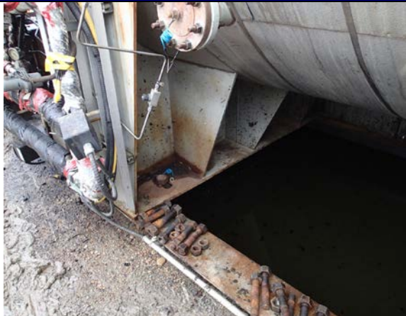
The vessel saddle sitting on the structural steel.
