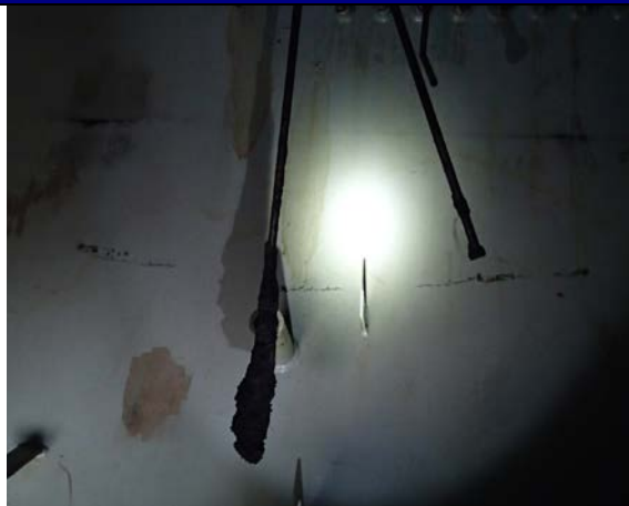
The bottom two sample lines that are plugged off.
