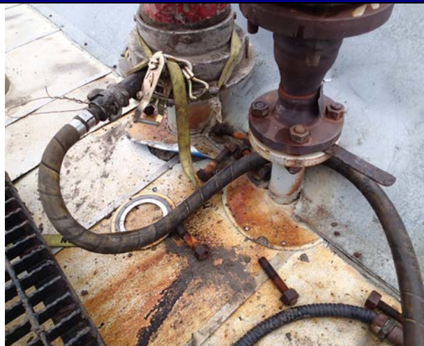
Cladding that requires repair on the top of the vessel.
