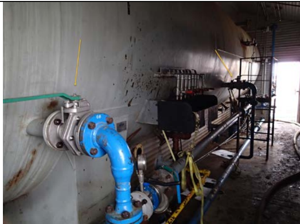
Desand outlet piping all the valves were removed except for the two 3" valves with arrows pointing at them.
