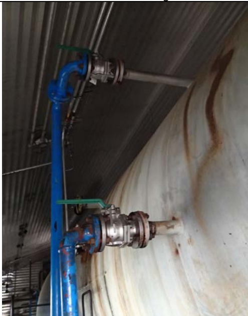
The two desand firetube valves that were not removed for inspection.
