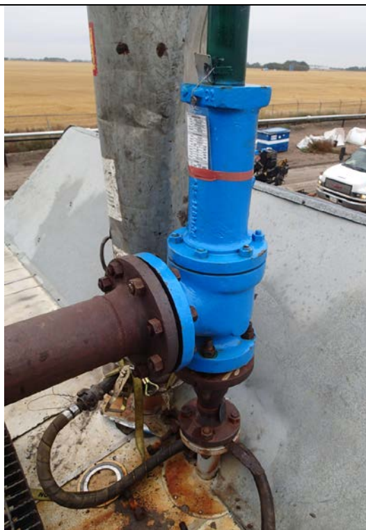
PSV attached to the vessel.
