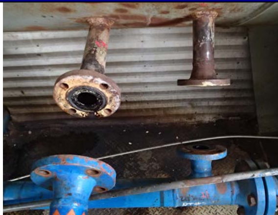
The desand inlet and outlet valves removed for flange face evaluation.
