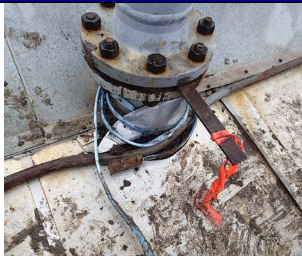
Cladding that requires repair on the top of the vessel.
