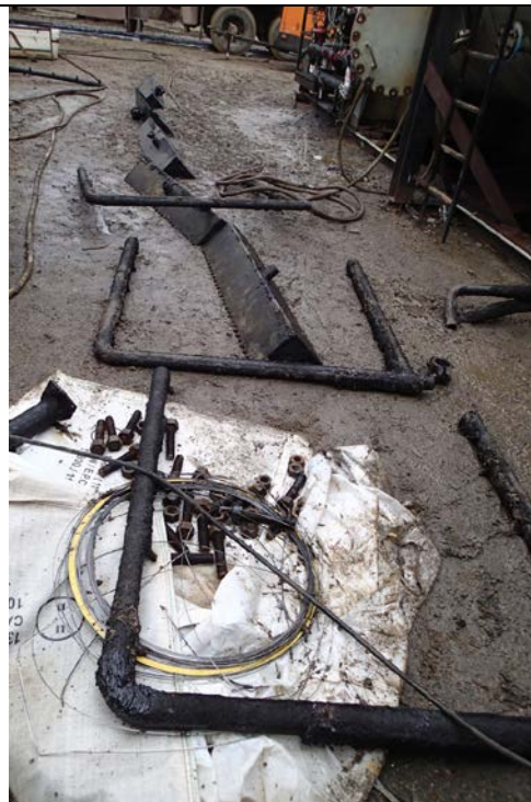
The sand pans and desand piping removed from the vessel.
