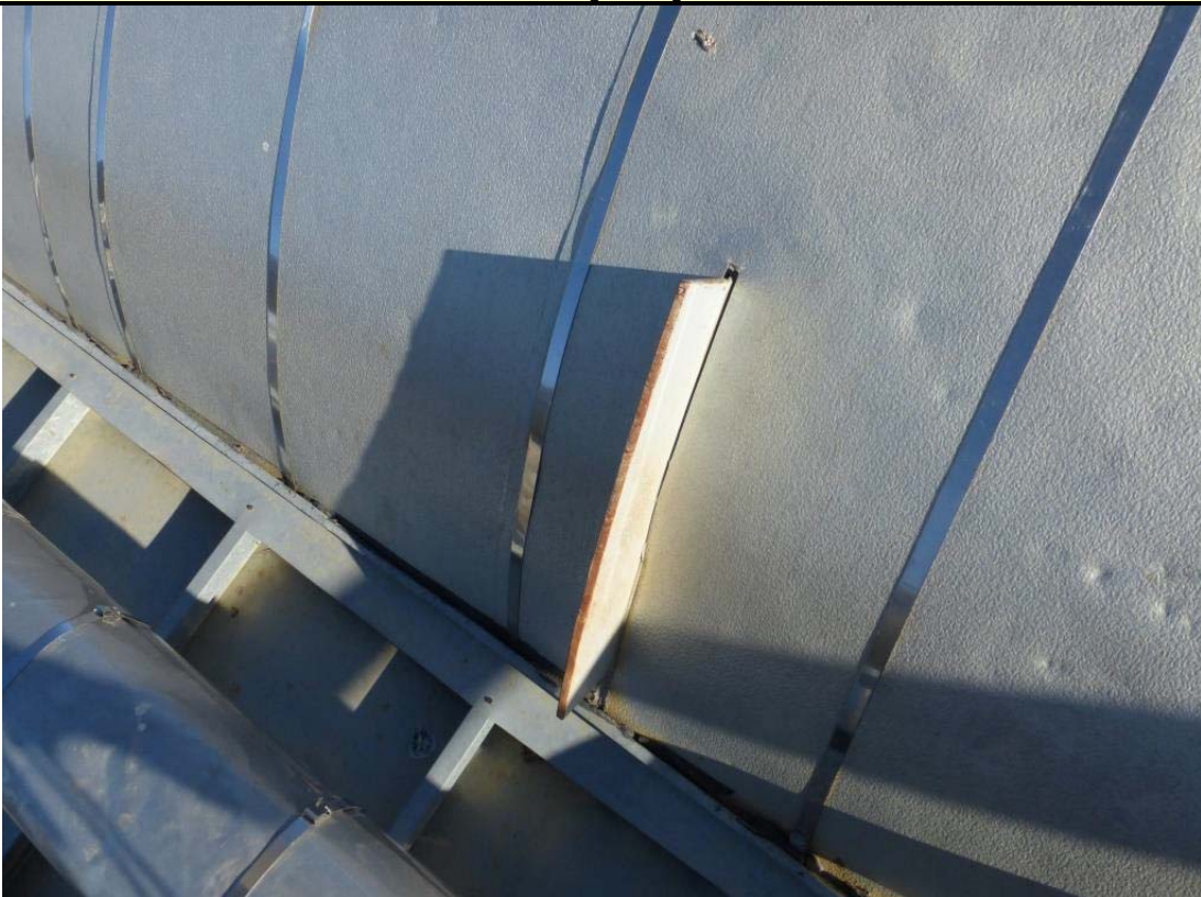
Insulation Penetration with no sealant
