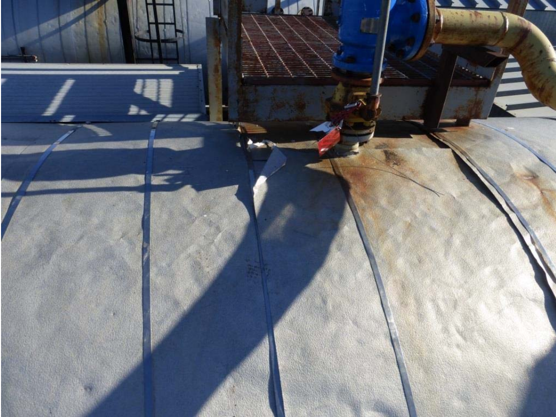
Cladding Damage
