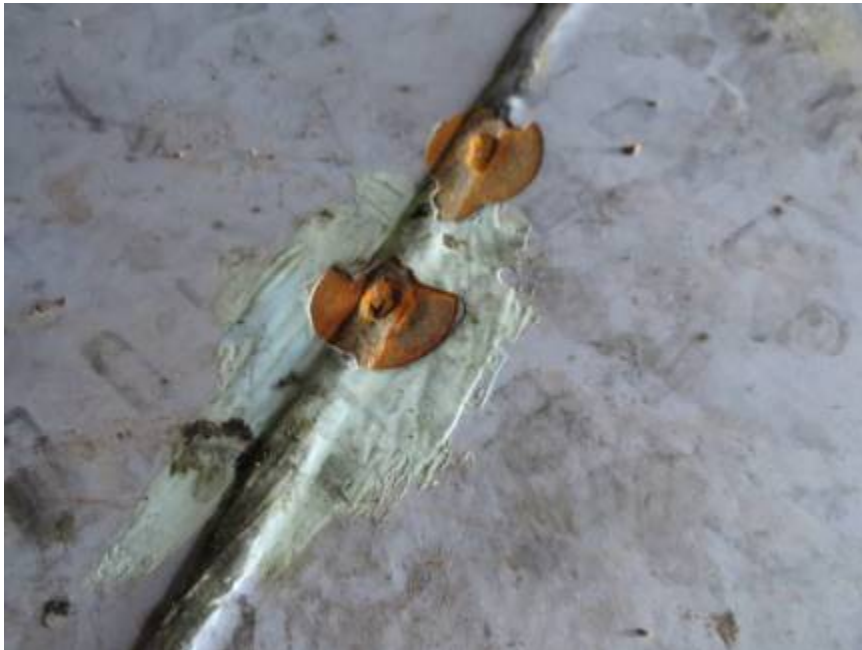
Photograph #11: Bottom Plate Weld Corrosion
