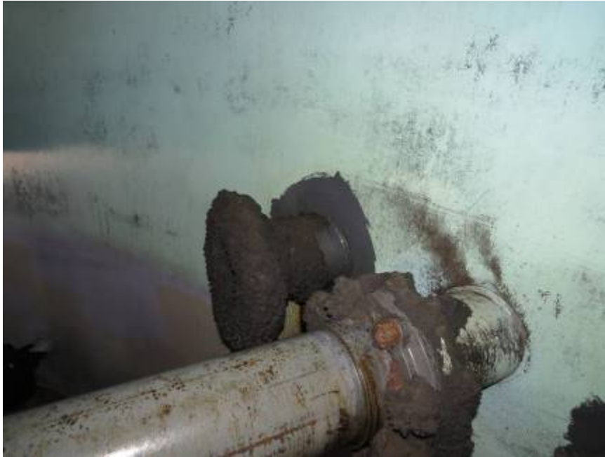
Photograph #32: Internal Nozzles
