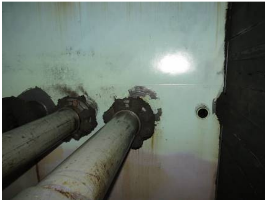
Photograph #31: Internal Nozzles
