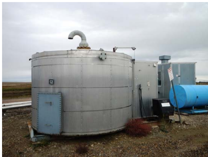
PRODUCED WATER TANK
